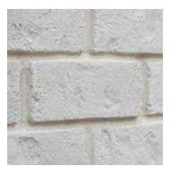
The most common grout technique is a standard or raked joint. This is what you typically see with brickwork, for example. The grout is evenly applied around the edge of each brick. When finished, the
