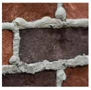
For a more old-world look, choose overgrouting. This technique uses a much heavier grout seam.
